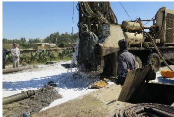
Borehole drilling in progress
